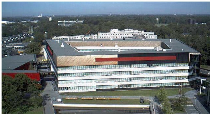
Figure 4.15: The east side of Carré building
